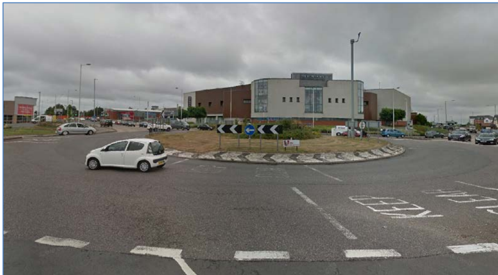
Figure 4 - Westwood Roundabout (A256 / A254)
